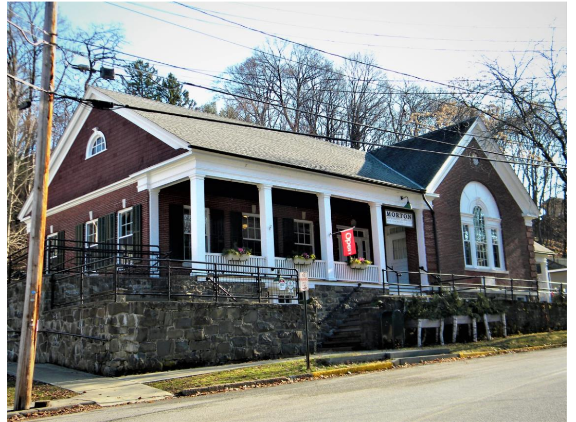
Morton Memorial Library & Community House (Rhinecliff, NY) [1908]
